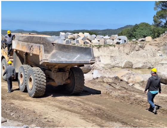
#Quarry Operations: Owned by nearby processor. Lease of around 100ha of Land
